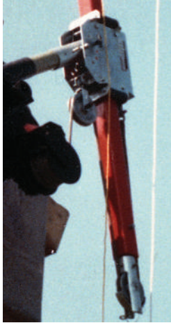
Winch line connects to mast base to raise conductors and provide working clearances for operator.
