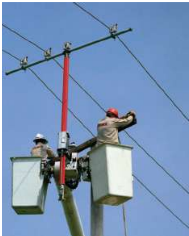
Wireholders latch easily from bucket with hookstick. 12" Epoxirod link insulates each latch-release lanyard.
